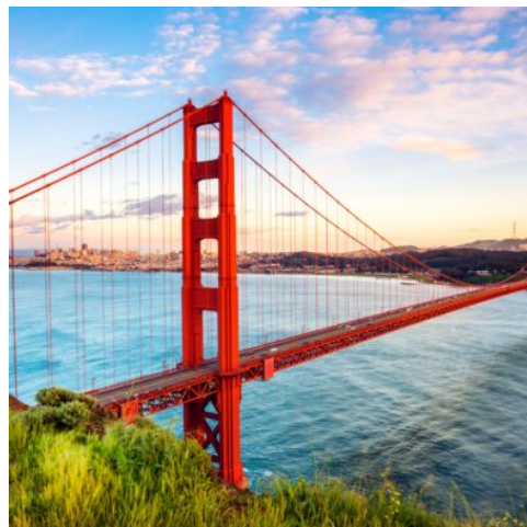
San Francisco - Golden Gate Bridge
